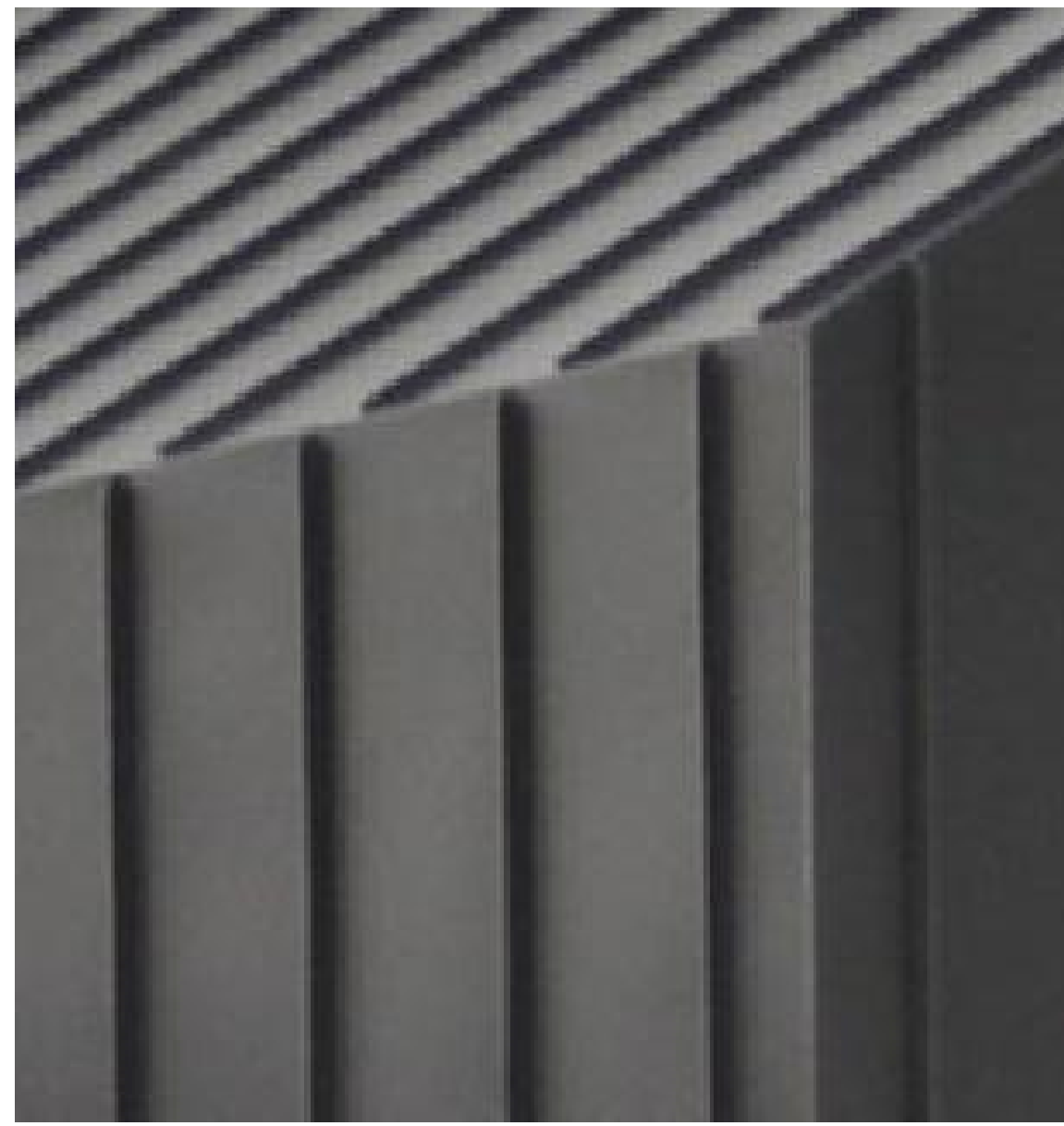
EF05 METAL ROOF TYPE 2: STANDING SEAM
